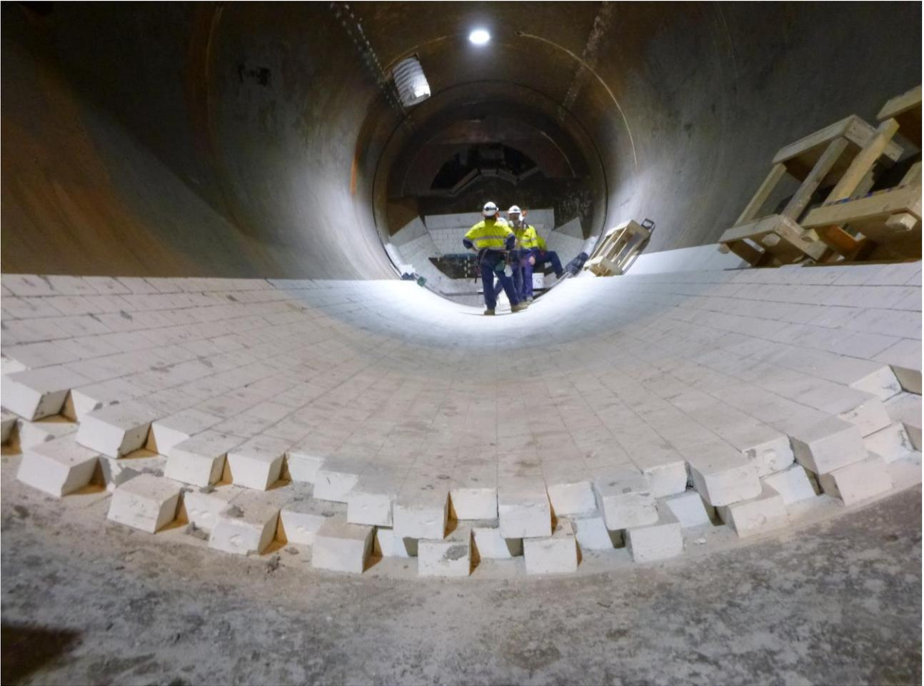
Furnaces re-bricked during the shutdown are lined with multiple layers of custom produced bricks to withstand the temperatures, up to 1200 degrees Celsius, generated during the smelting process.
