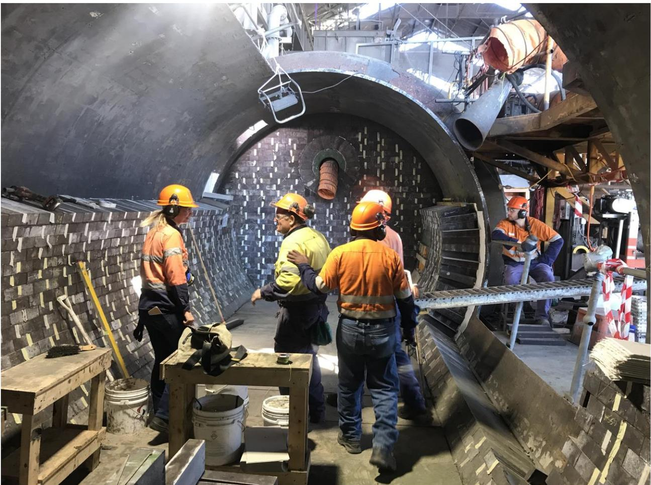
Re-bricking underway in the anode furnace during the \$30 million Copper Smelter shutdown in March and April.
